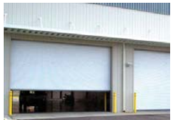
With Cornell windloaded doors, new Lewis Bear Facility survives
