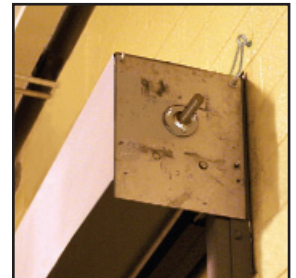
Door is prepped for new M100 operator.
