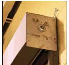
Door is prepped for new M100 operator.
