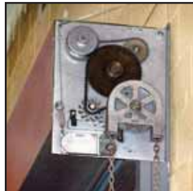
Conventional fire door chain operator, governor and complicated drop out mechanism.
