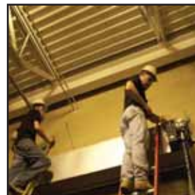
Installers reattach existing fusible link to new operator.
