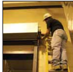
Existing operator, governor and dropouts are removed and discarded.
