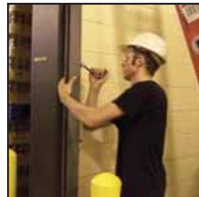
Installer prepares to mount the floor level pull cable.
