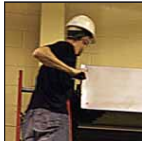
Installation of M100 Retrofit unit. Spring tension of door is temporarily relaxed.
